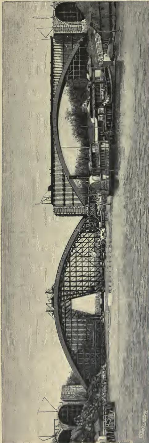
The 510-feet Span Steel Arches of the New Harlem River Bridge, New York, during construction.
