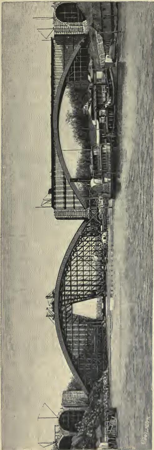
The 510-foot Span Steel Arches of the New Harlem River Bridge, New York, during construction.
