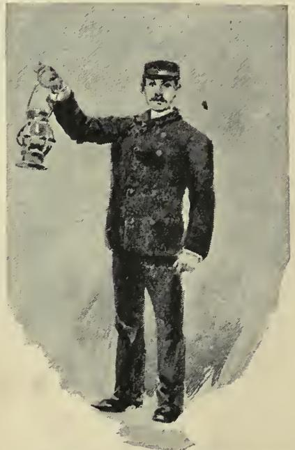
A lamp raised and lowered vertically is the signal to move ahead.
